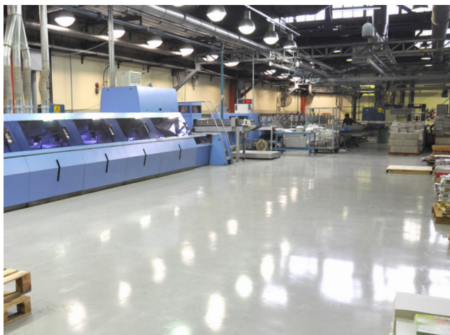
FERROPUR SL® + FERROPUR 70® (JOINTLESS)
