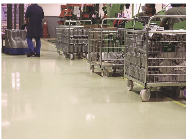
FERROPUR SL® + FERROPUR 70® (JOINTLESS)
