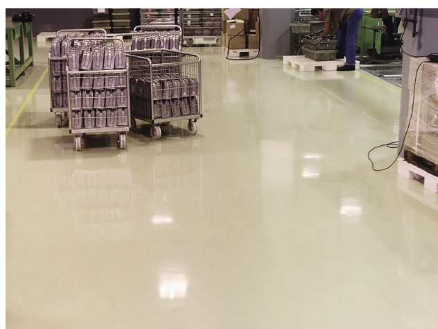
FERROPUR SL® + FERROPUR 70® (JOINTLESS)
