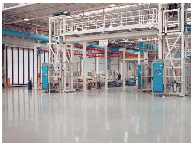
FERROPUR SL® + FERROPUR 70® (JOINTLESS)
