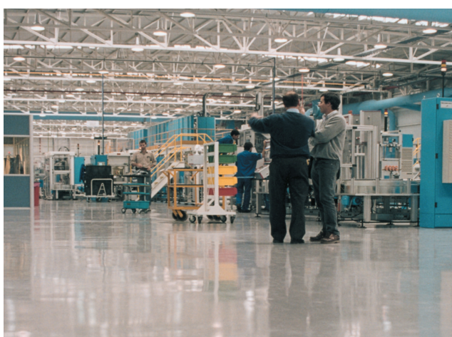
FERROPUR SL® + FERROPUR 70® (JOINTLESS)
