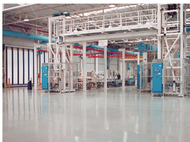
FERROPUR SL® + FERROPUR 70® (JOINTLESS)
